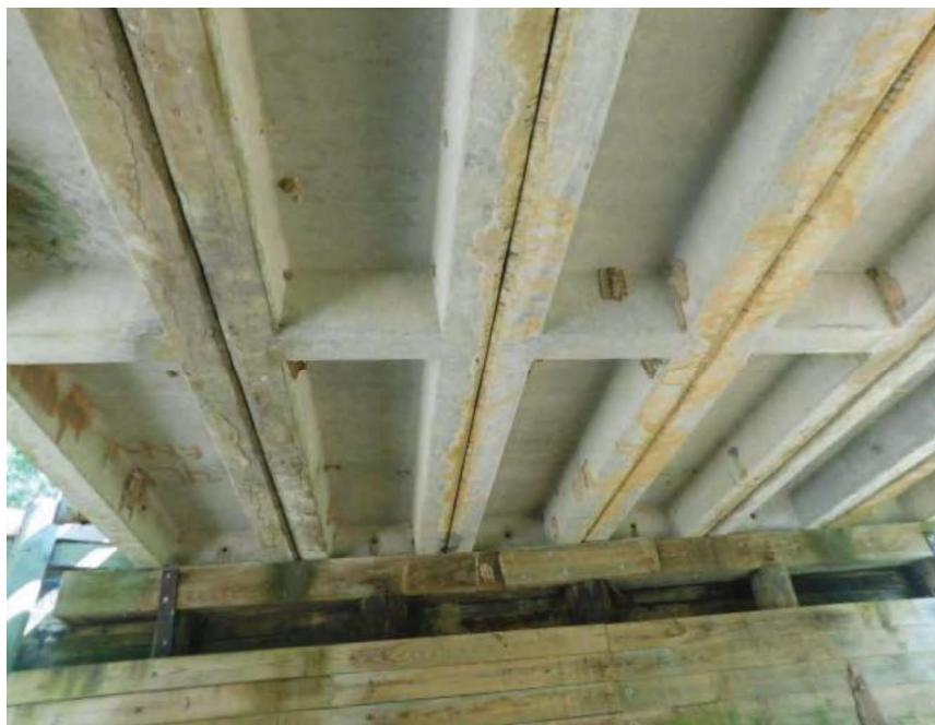
BOTTOM DECK SPAN 2
