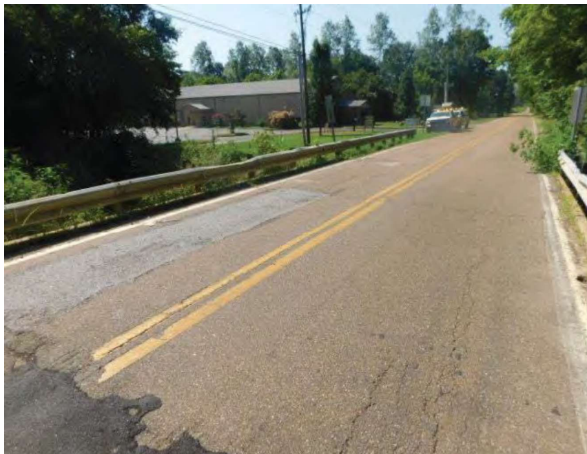
VIEW ACROSS TOP OF DECK
